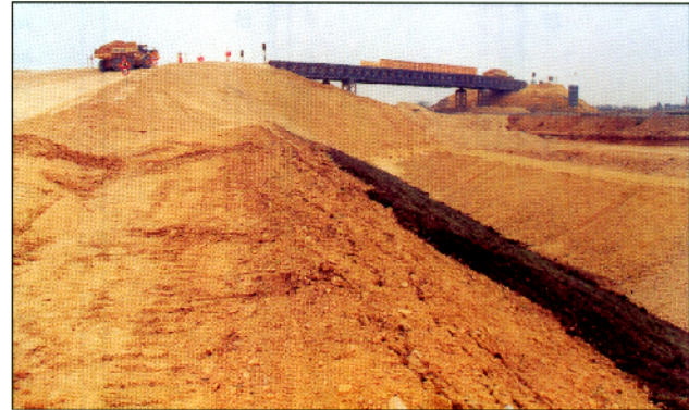
Above: The temporary bridge at Hook Moor
