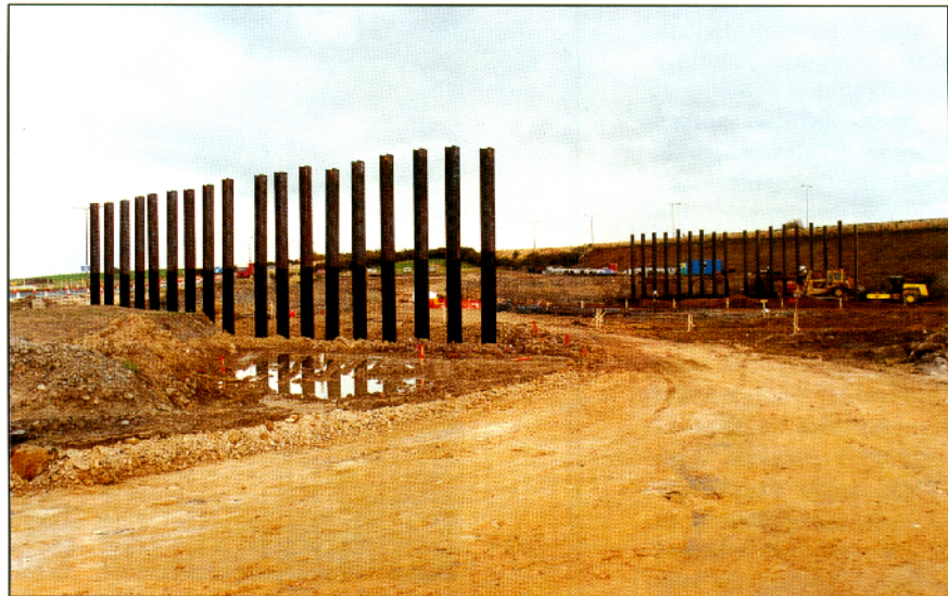
Above : Foundation Works at Rothwell High
