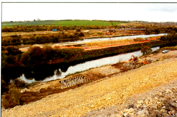
Left: Piling for the Aire Valley Viaduct
