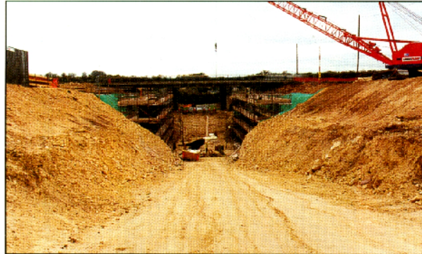
Construction of Lofthouse Lane Bridge, Aberford
