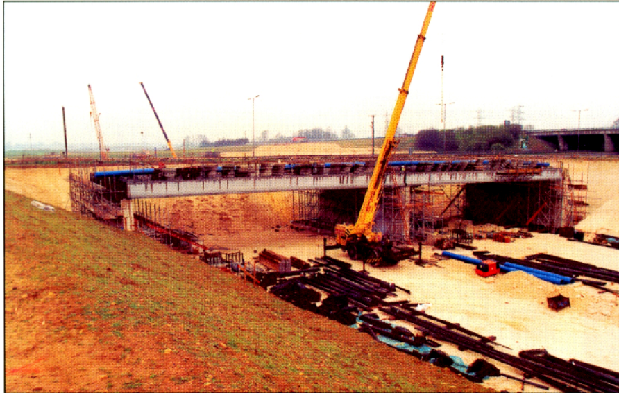
Above: Bramham Crossroads south bridge
