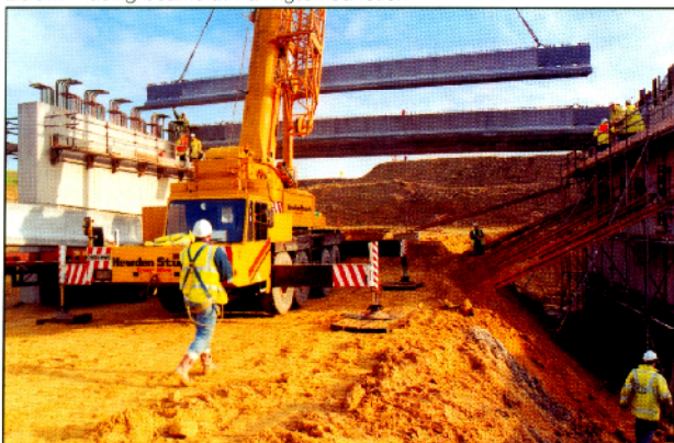
Below: Placing beams at Parlington Junction
